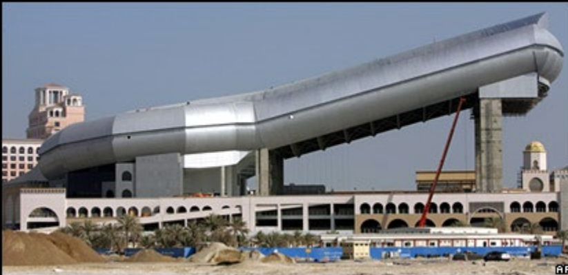
Ski Dubai, 85m high by 80m wide, has to cope with average outside winter temperatures of 25C and summer temperatures soaring above 40C.
